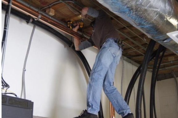
Keith Peterson installs the brackets for the new 3-1/8" transmission line
