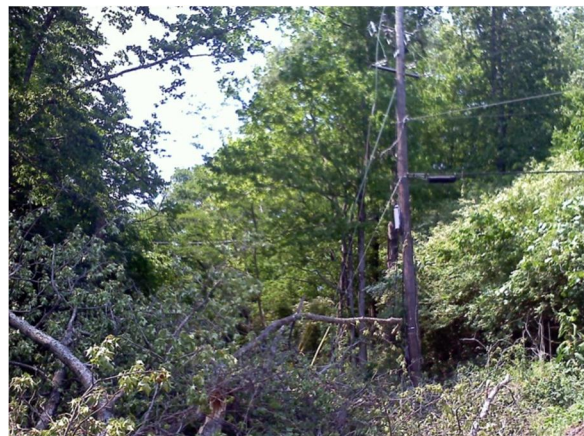
A tree across the road and tangled in power lines blocked access to the WDJC-FM site
