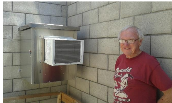
KBRT transmitter engineer Fred Folmer with the temperature-controlled, weatherproof translator cabinet at tower #1.
