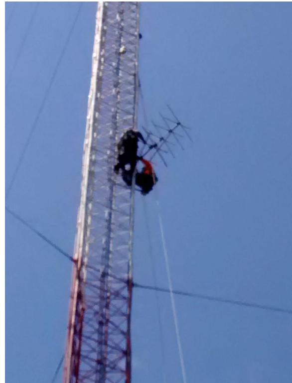
Figure 6 - The California Crew mounting the translator antenna at Red Mountain.
