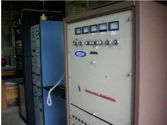
The WDCX(AM) ND-5 (L) and 315R (R). A low-time ND-5 will soon replace the 315R.
